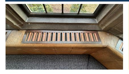
The heaters lining the benches in the Children's department have had pieces of oak installed underneath the grates to create a buffer between the radiator and the copper grate its self. While this strategy has minimized most of the heat, additional measures are being researched including replacement of the grates to a different material, in order to meet safety guidelines.
