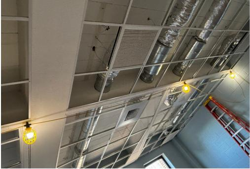
**Study Room Project:** The construction of the Study Rooms in the Cooper Building is still underway. Floor leveling, painting, header installation, drop ceiling grid, and HVAC have been installed. Remaining phases include electrical and installation of the study room walls and doors. Furniture and technology will also be acquired for each study room.
